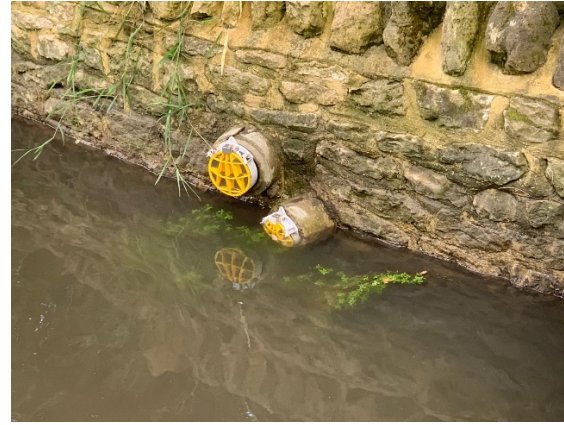
Road gully outlets leading directly into Halls Lane Non-return valves fitted July 2024
