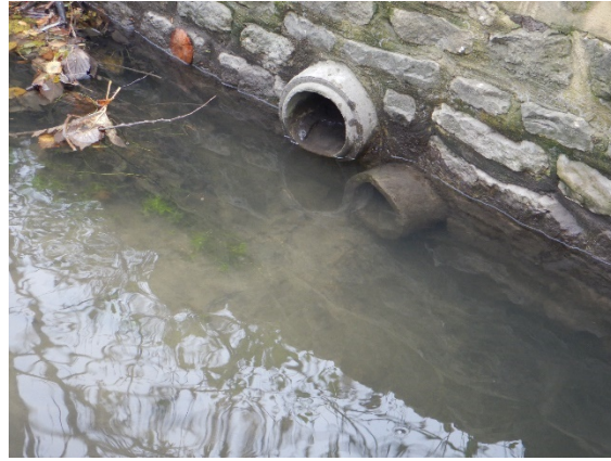
Road gully outlets leading directly into Halls Lane Non-return valves fitted July 2024
