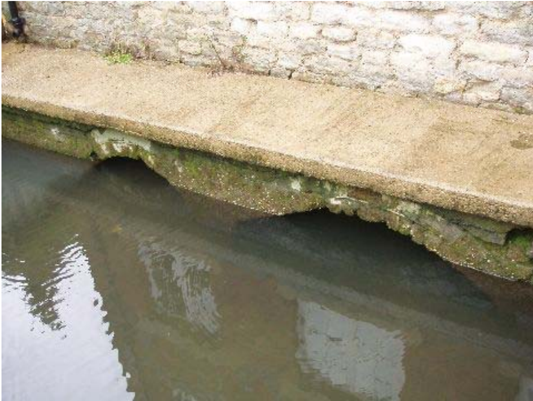
Wantage Mill - Twin masonry arch culverts under mill has trash screens on downstream end
