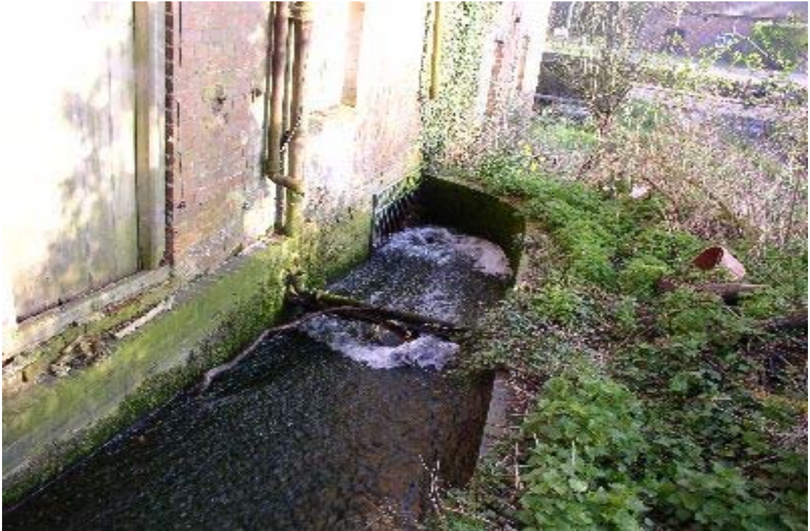
Dandridges Mill - Weir and side mill by-pass channel.
