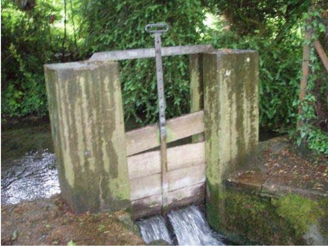
Concrete side sluice with timber lifting gate – the leat, Wantage
