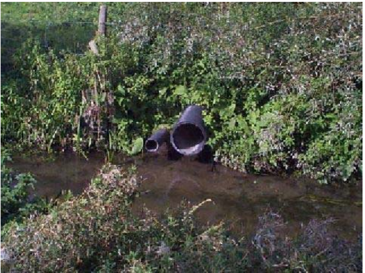
Lower Mill, East Hanney - Black plastic pipes feeding mill bypass channel.
