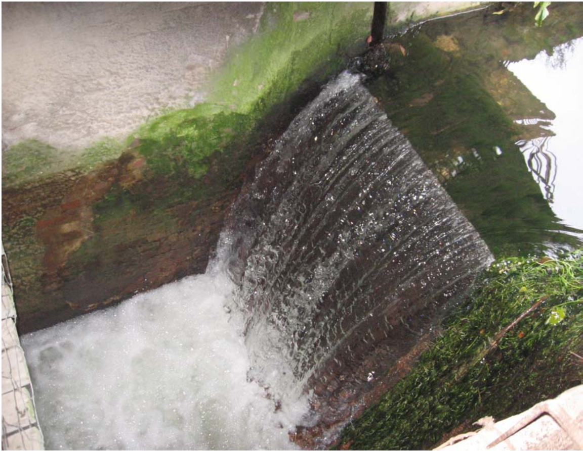
Lower Mill, East Hanney – Fixed crest weir.
