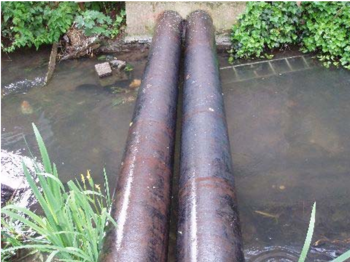
Twin service 600mm pipes across the Letcombe Brook - Wantage
