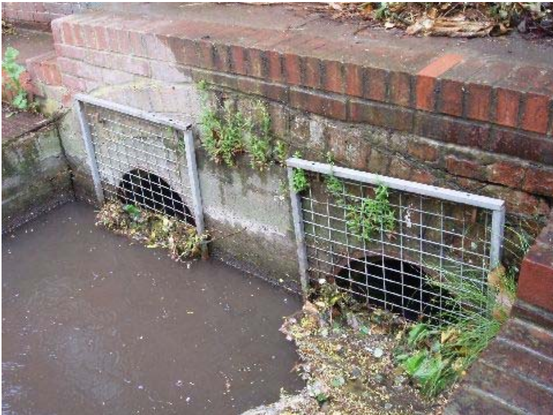
Wantage Mill - Twin masonry arch culverts under mill has trash screens on upstream end
