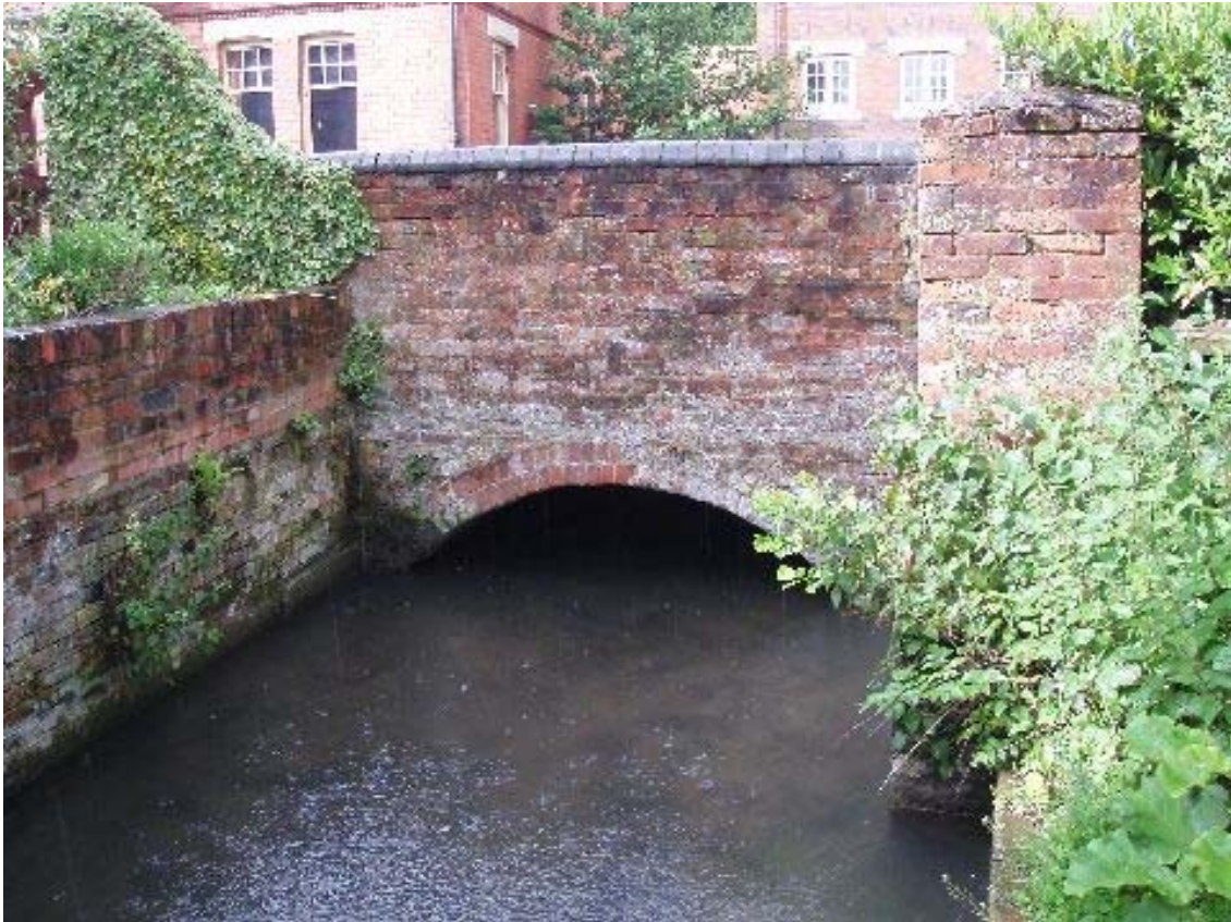
Mill Street Road bridge
