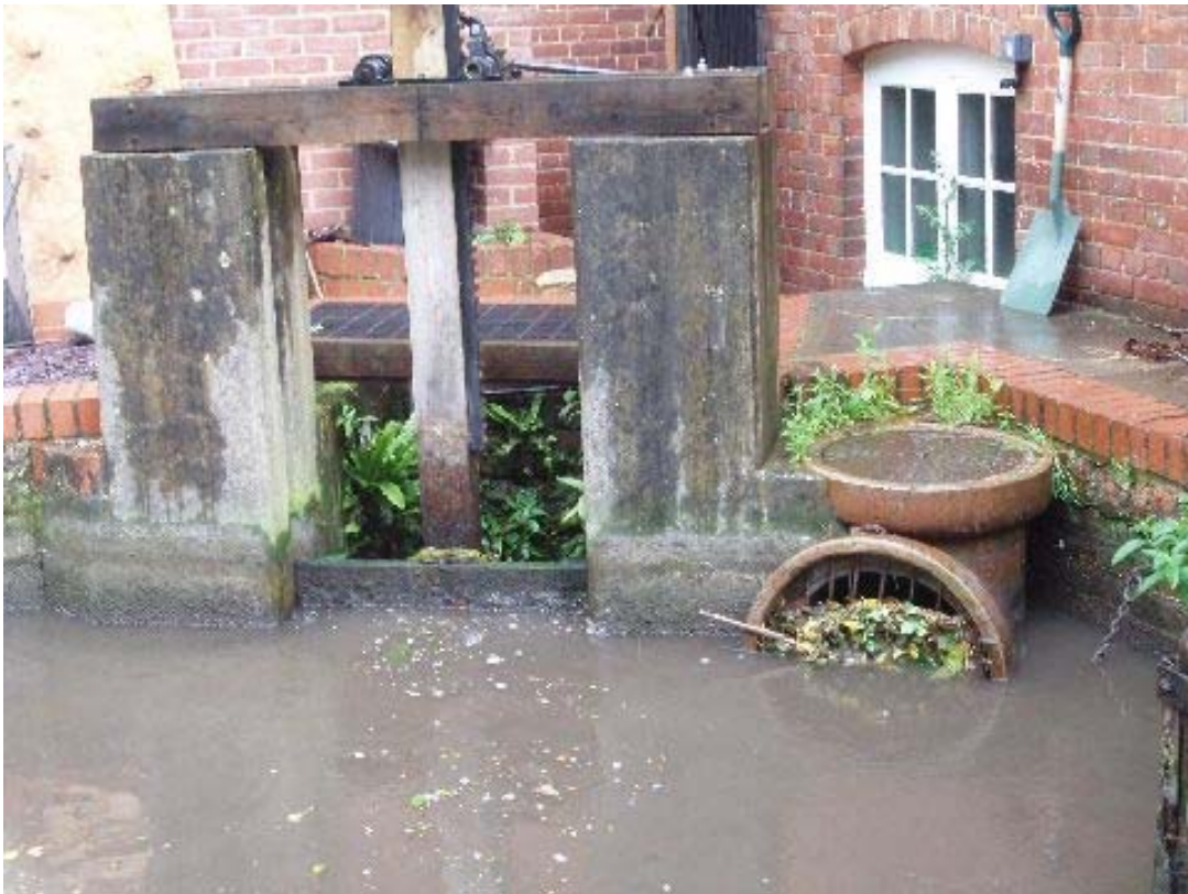
Wantage Mill, (upstream) - Side sluice (bypass for mill control) concrete channel sides with timber lifting gate in timber frame also has 500mm clay pipe to allow extra capacity.
