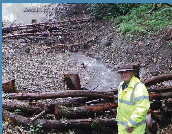
Figure 16.2 Leaky dams
