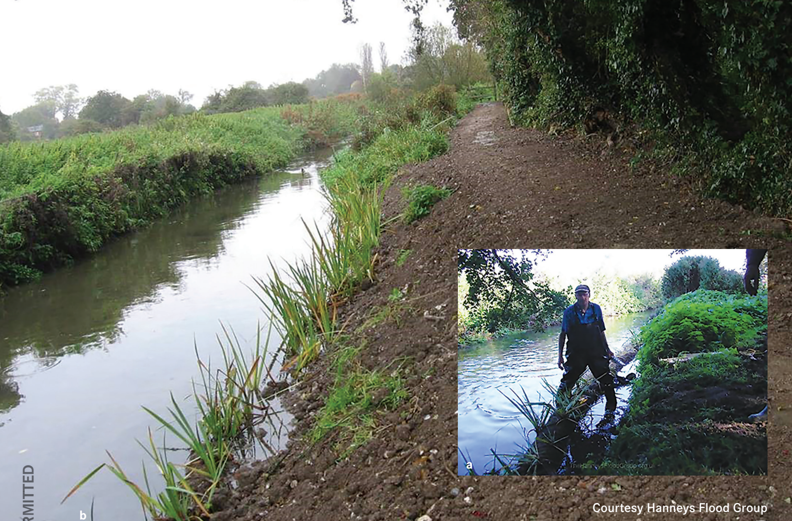
Figure 17.1 Installing coir rolls (a) to provide stabilised toe to reinstated flood embankment slope (b) and to encourage waterline vegetation
